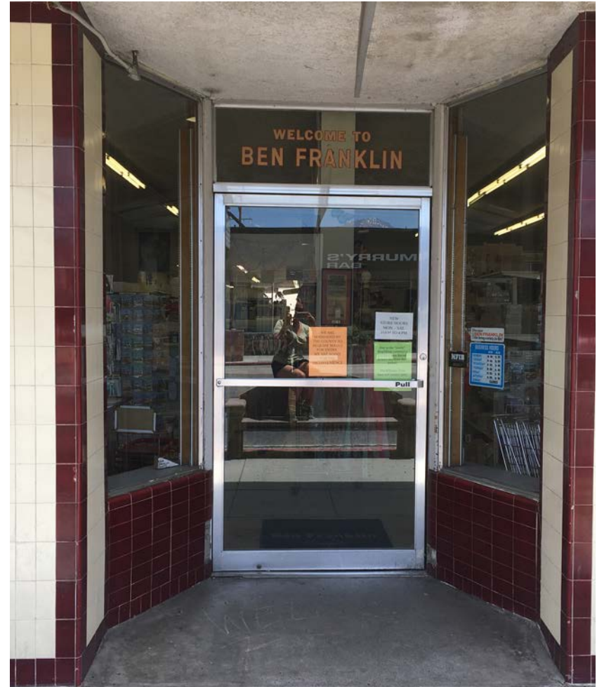
Recessed building entrance in Bishop, CA
