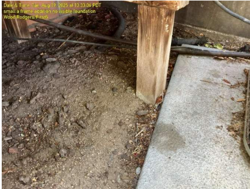
Photo 24 – Showing post in contact with earth and no apparent foundation
