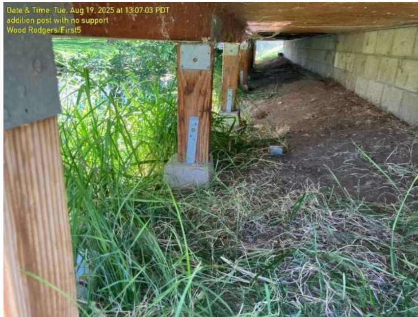
Photo 16 – Creek encroaching on post foundations.
