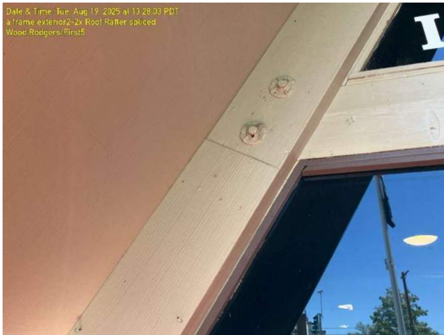
Photo 3 – At West side roof gable, roof rafter splice just below collar tie connection.
