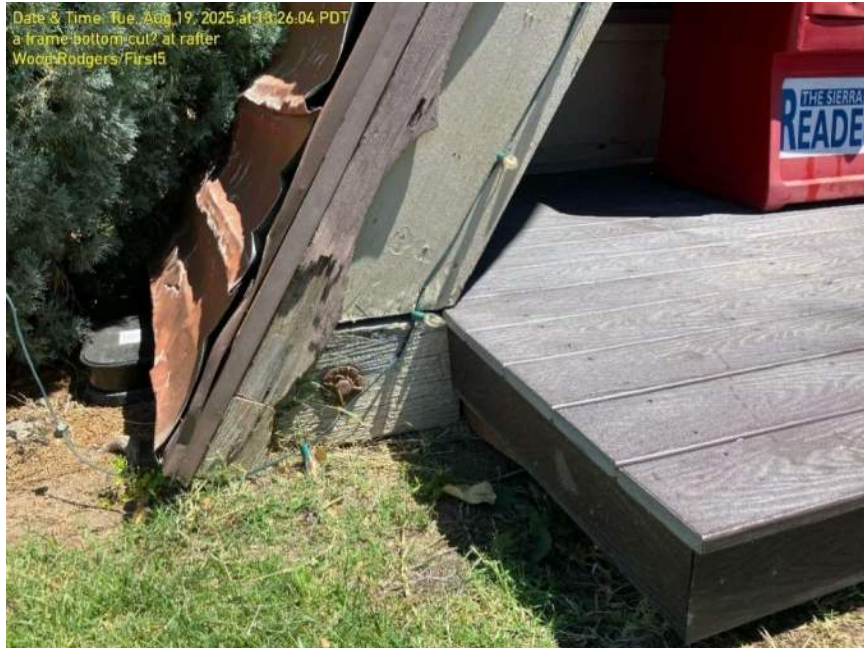
Photo 9 – Northwest corner of first floor foundation. No ventilation.
