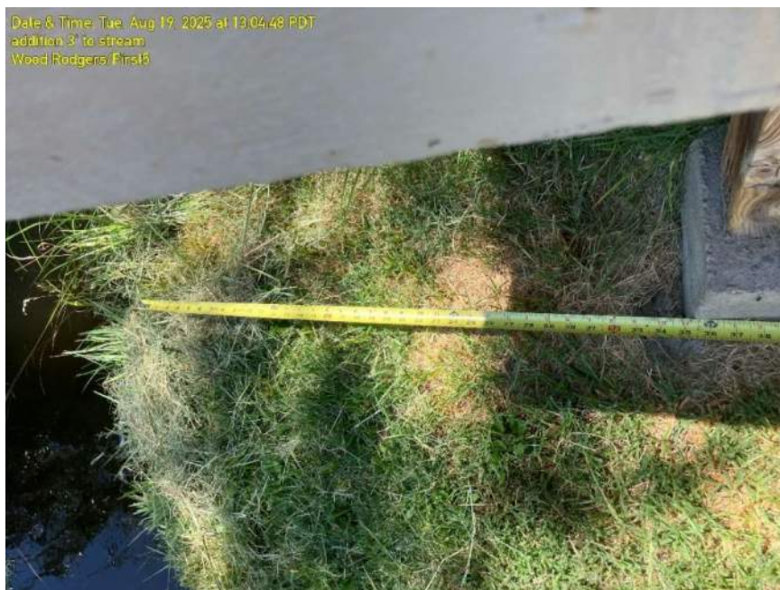
Photo 15 – Creek within three feet of the post foundation.
