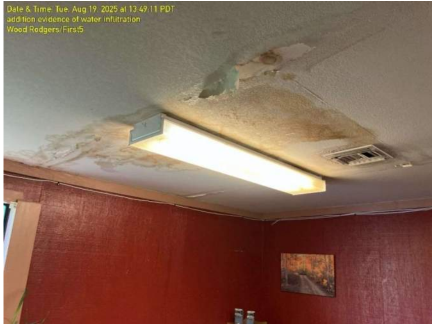
Photo 17 – Visible signs of possible roof leak.
