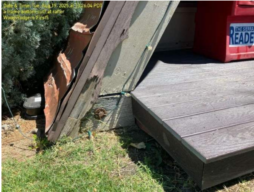
Photo 7 – Northwest corner of first floor to rafter connection, one (1) bolt and floor joist cut.
