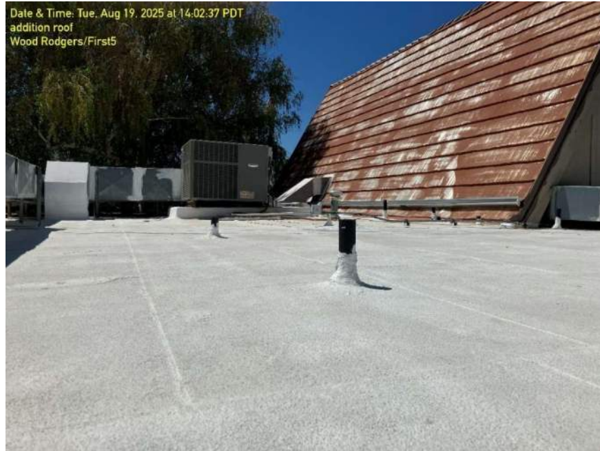
Photo 19 – No apparent roof slope or drainage.
