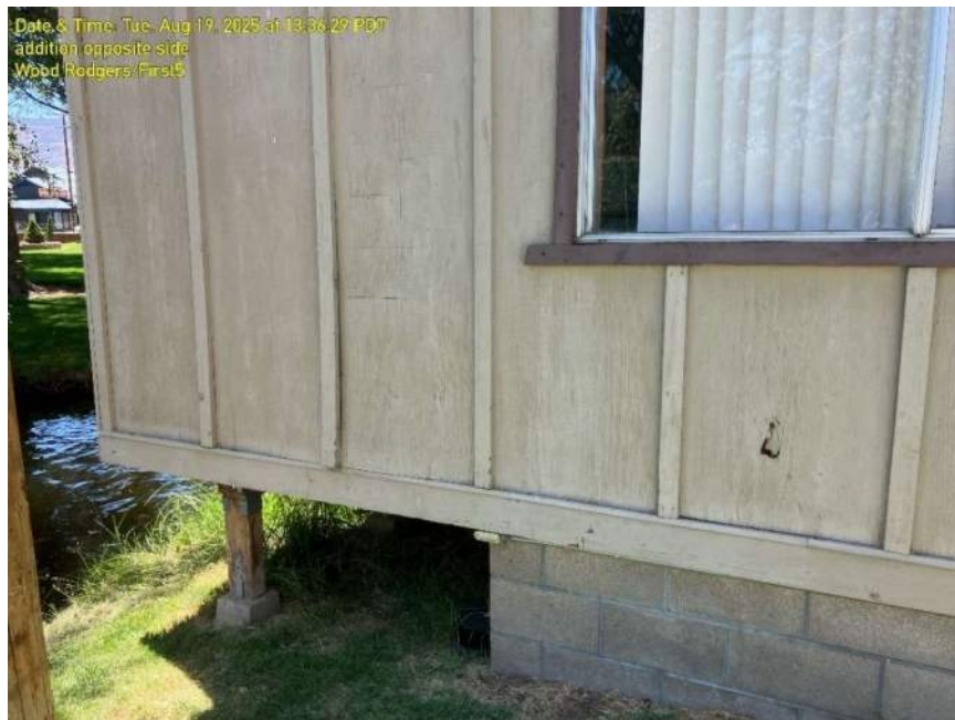
Photo 23 – No visible venting of First floor level on West side of Addition
