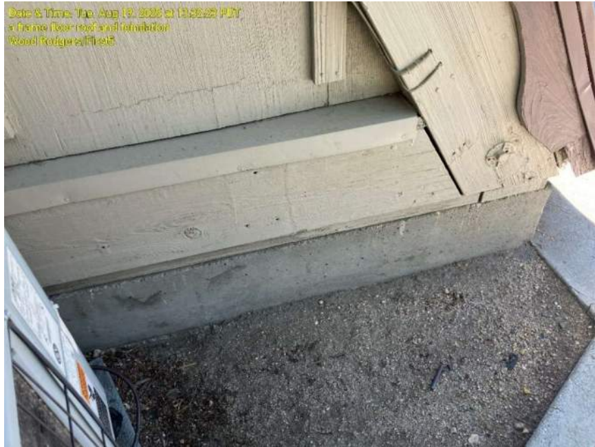
Photo 11 – Northeast corner of first floor foundation. No ventilation.
