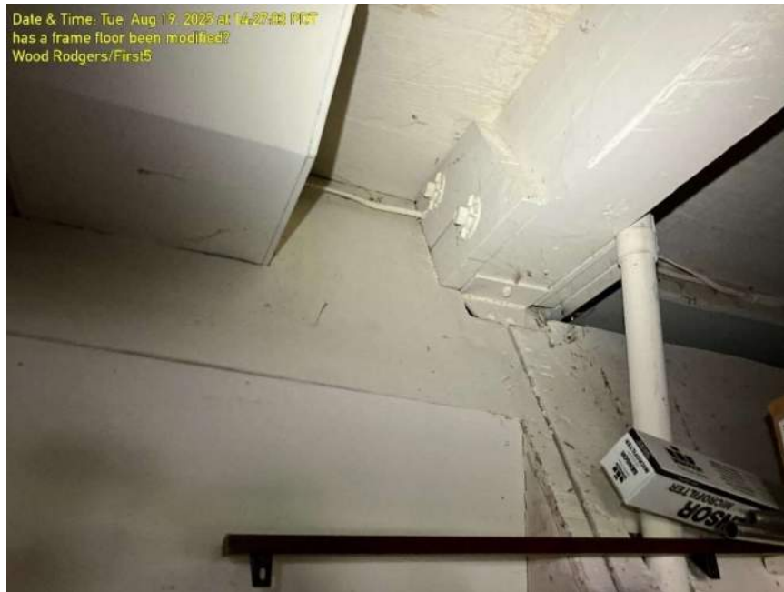
Photo 20 – 6x12 Roof Joist connection at A-Frame Floor.
