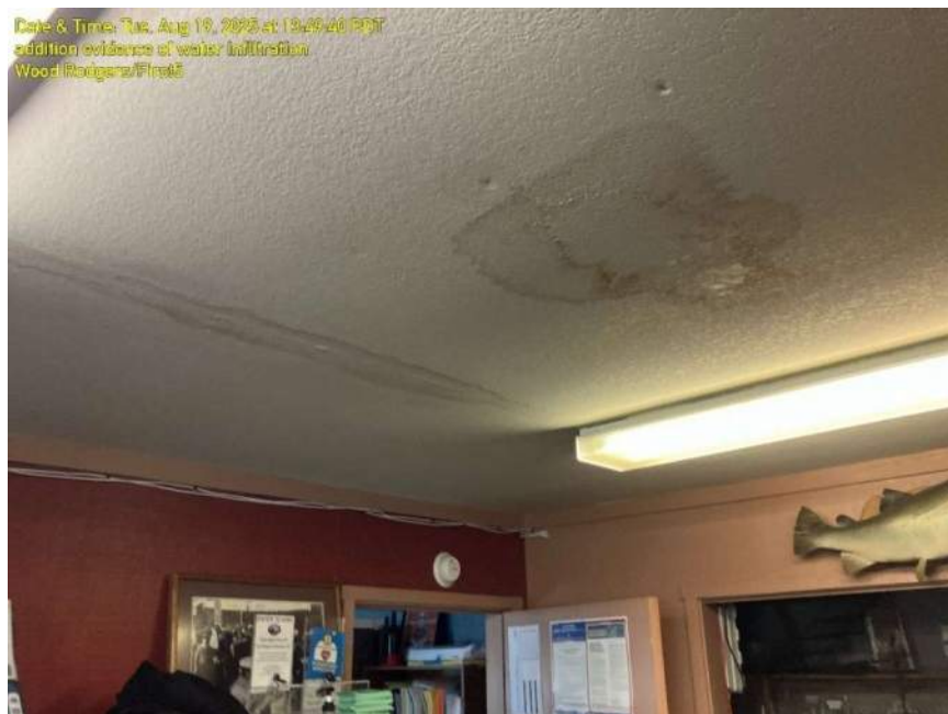
Photo 18 – Visible signs of possible roof leak.
