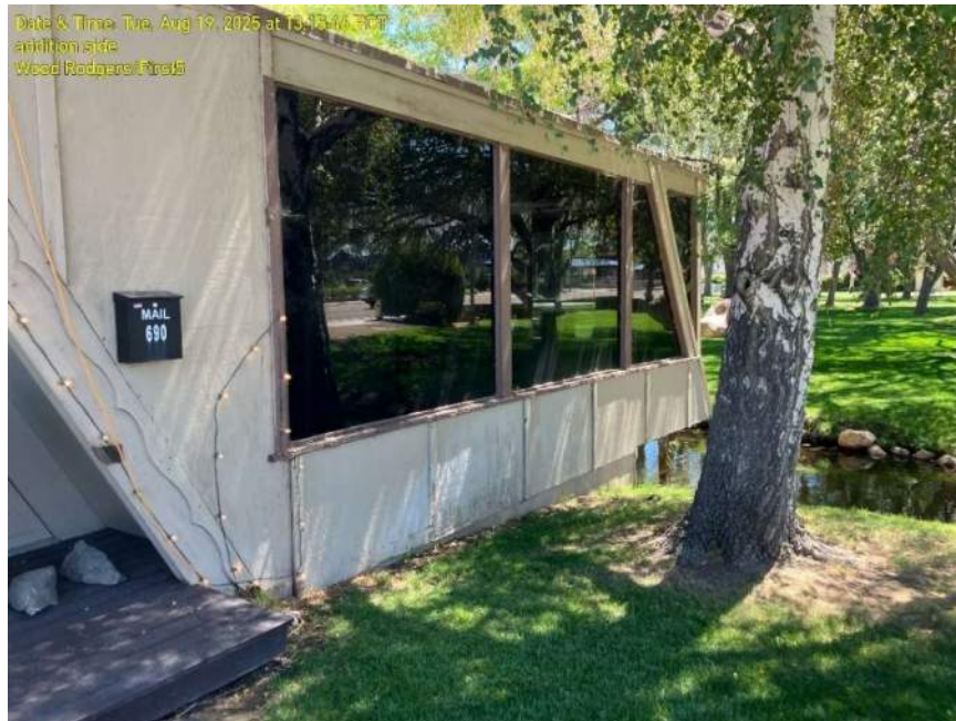
Photo 22 – No visible venting of First floor level on West side of Addition
