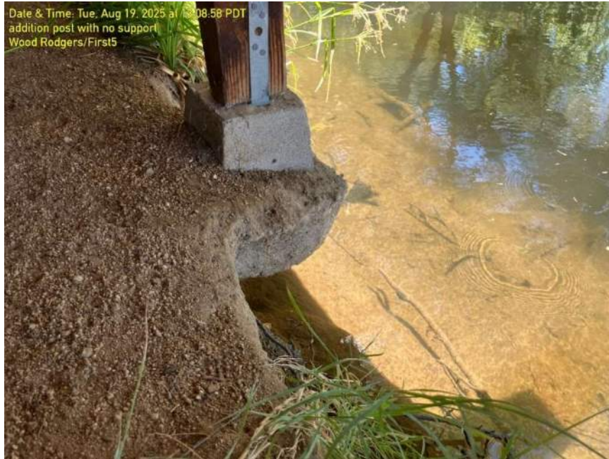
Photo 14 – Soil erosion by Creek under concrete footing
