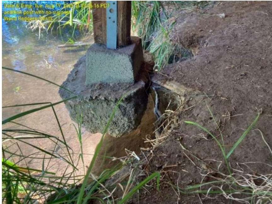
Photo 12 – Concrete footing undermined by Creek.
