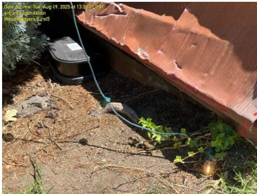
Photo 10 – North Foundation stem wall of first floor foundation. No ventilation.
