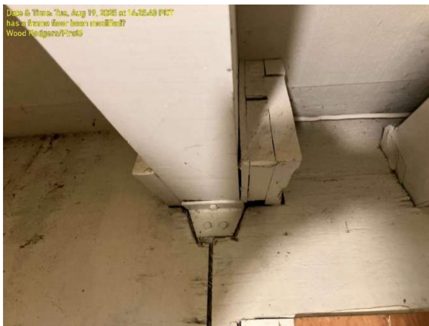
Photo 21 – 6x12 Roof Joist connection at A-Frame Floor showing additional members
