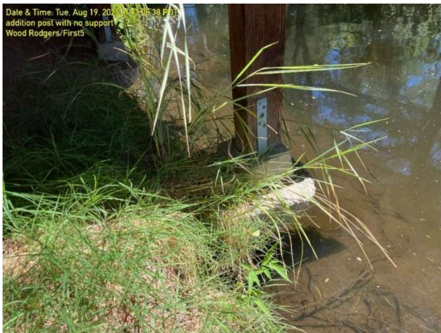
Photo 13 – Soil erosion by Creek under concrete footing
