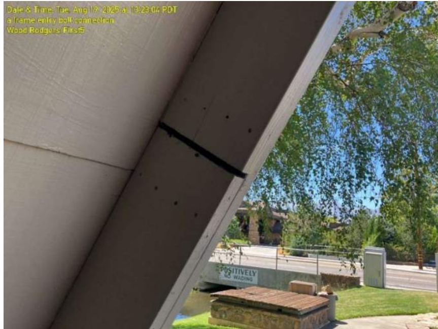
Photo 2 – At West side roof gable, roof rafter splice with larger separation.
