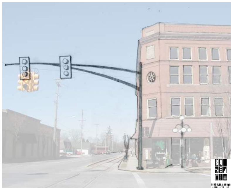
Example of mast arm traffic signal at Chicago Boulevard and Evans Street.
