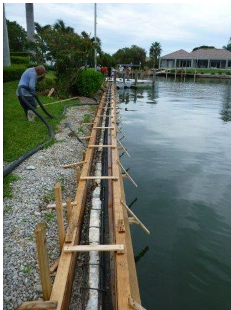
Framing and pouring of new (replacement) cap
