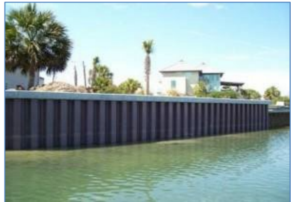
Vinyl Seawall with Concrete Cap
