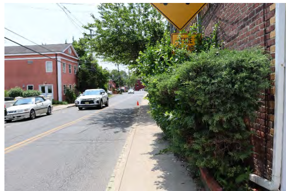
Existing Sidewalk Conditions – Note the narrow width in one location and encroachment in another.
