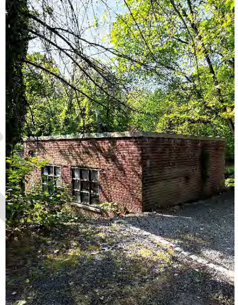
Image 3.5.2.12: Sparkill Pump House
